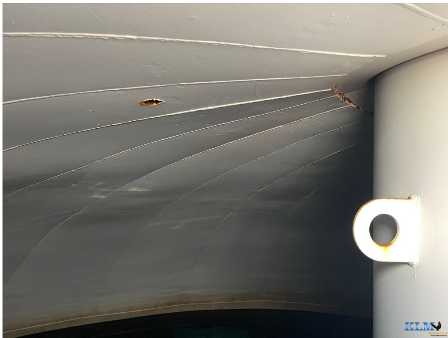
Photo No. 6 Roof conditions
