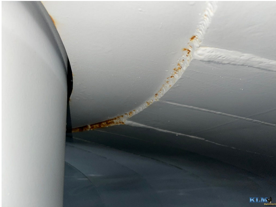
Photo No. 3 Interior roof conditions
