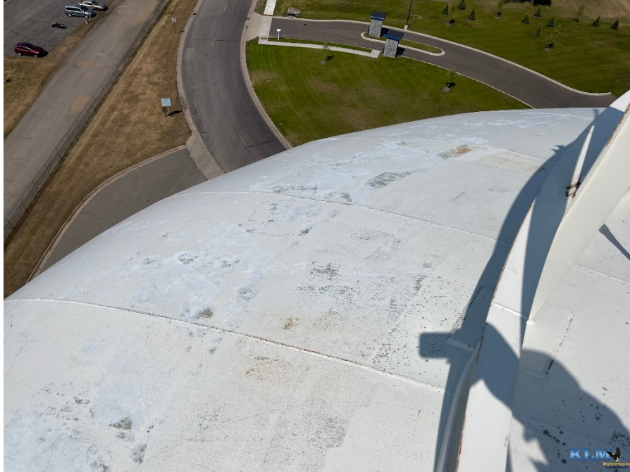
Photo No. 49 Roof coating conditions
