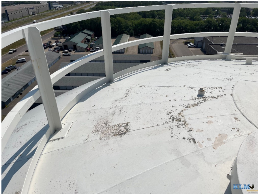
Photo No. 47 Roof conditions
