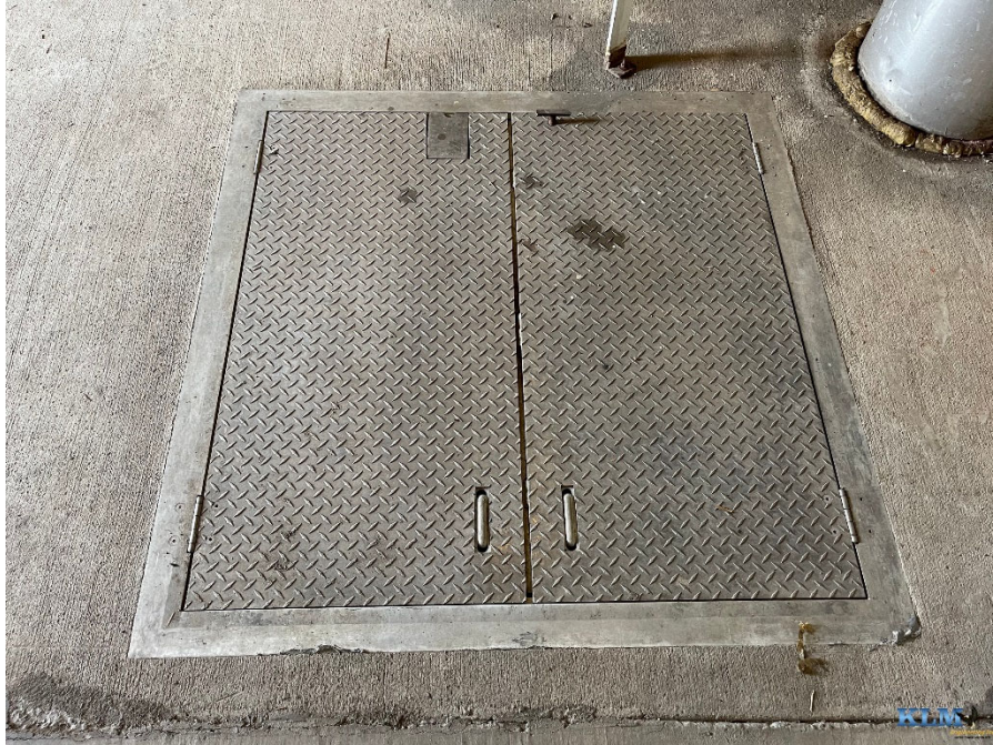
Photo No. 41 Valve pit manway
