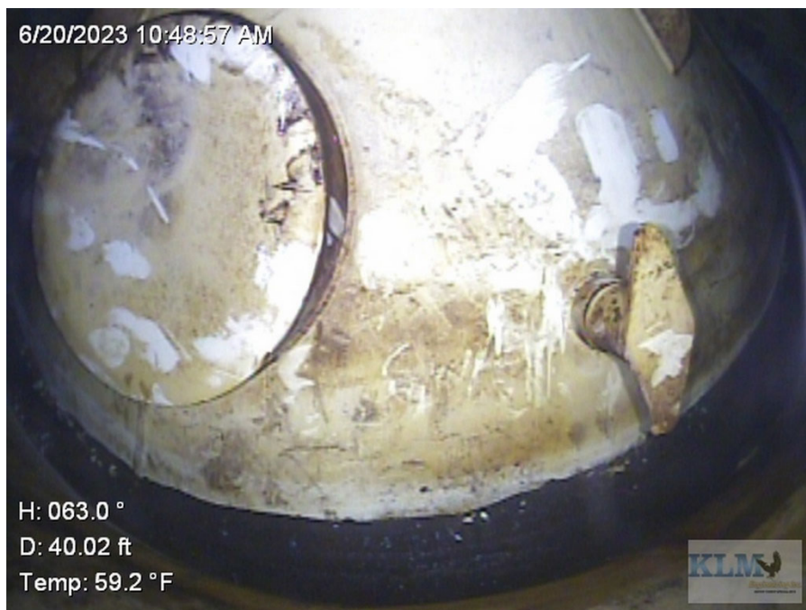
Photo No. 25 Bowl conditions with manway and drain plug visible
