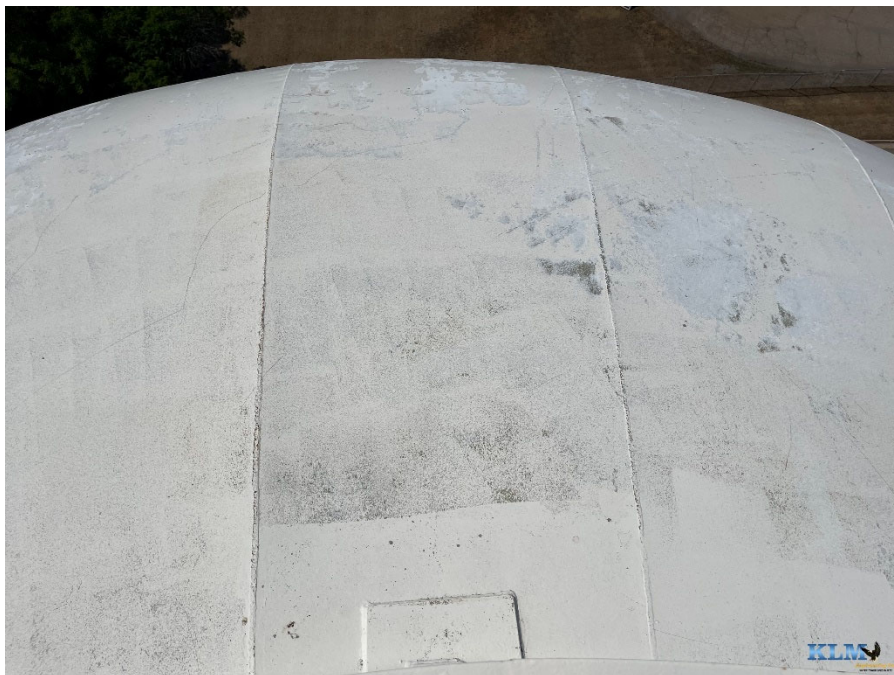
Photo No. 48 Roof coating conditions
