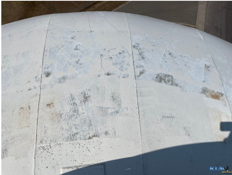
Photo No. 51 Roof coating conditions
