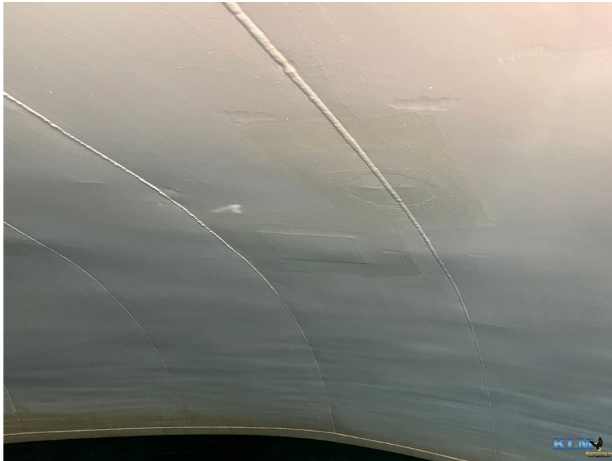
Photo No. 7 Roof conditions
