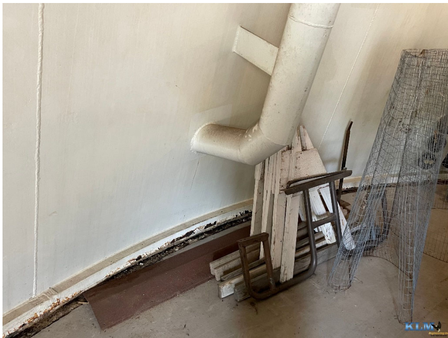
Photo No. 38 Base cone conditions
