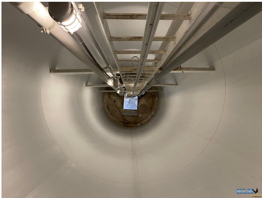
Photo No. 34 Pedestal conditions looking down at bottom landing
