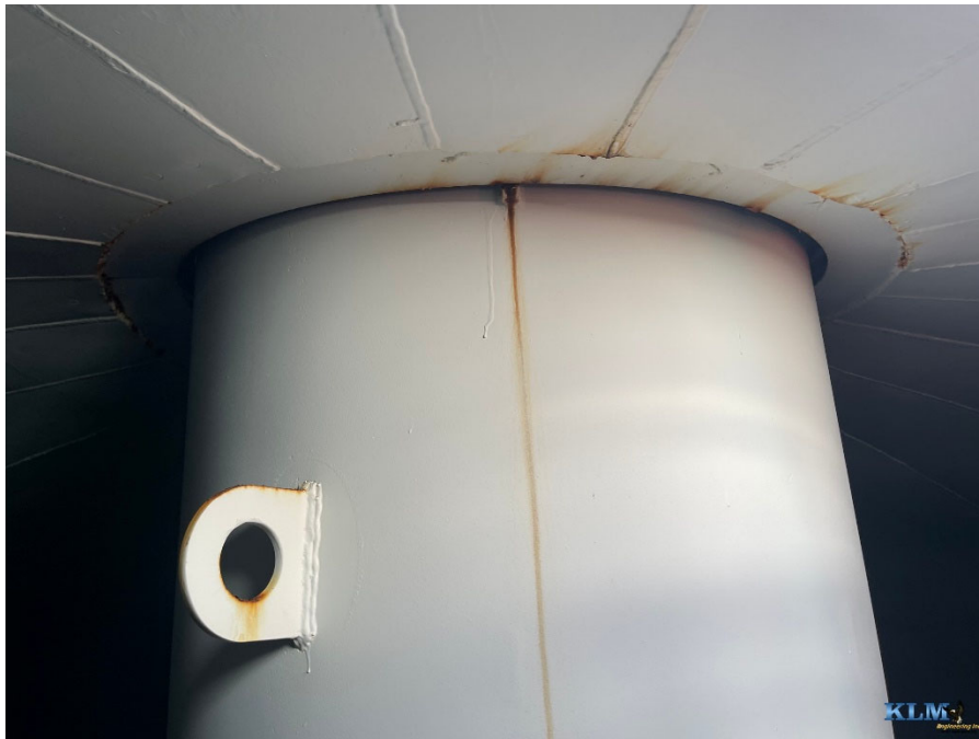
Photo No. 2 Top of drywell tube
