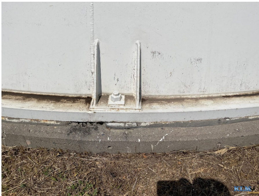
Photo No. 58 Typical foundation conditions
