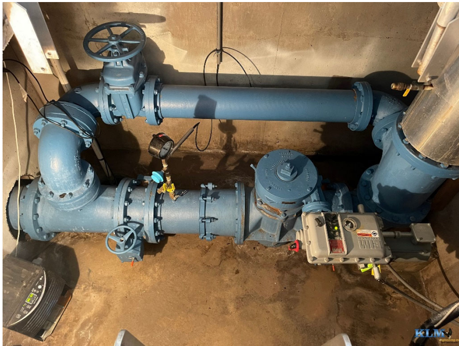
Photo No. 42 Valve pit conditions
