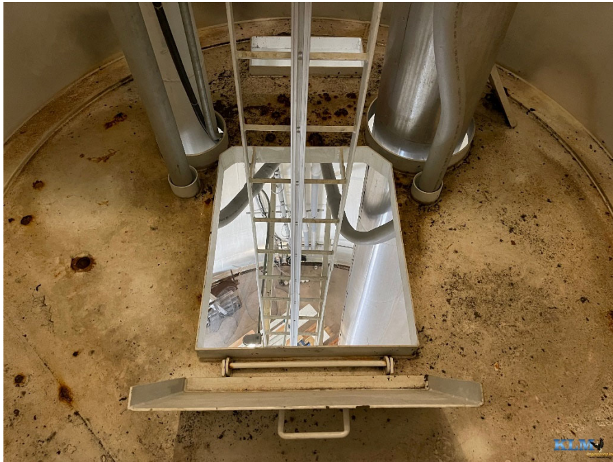
Photo No. 35 Bottom landing conditions
