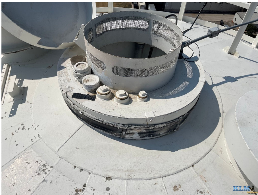
Photo No. 44 Drywell tube manway
