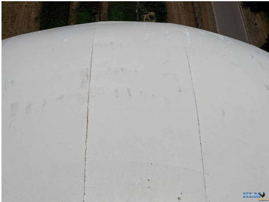
Photo No. 50 Roof coating conditions
