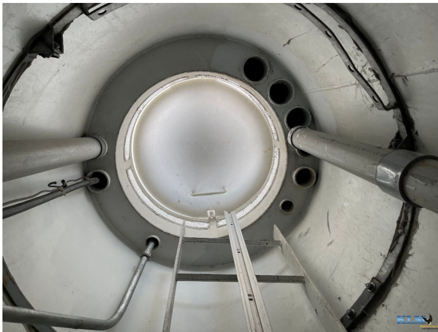
Photo No. 26 Top of drywell tube
