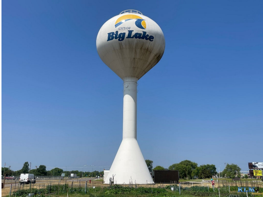
Photo No. 1 Overall view of tower
