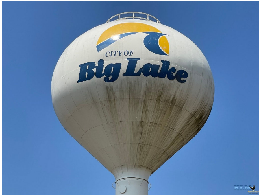
Photo No. 53 Water compartment
