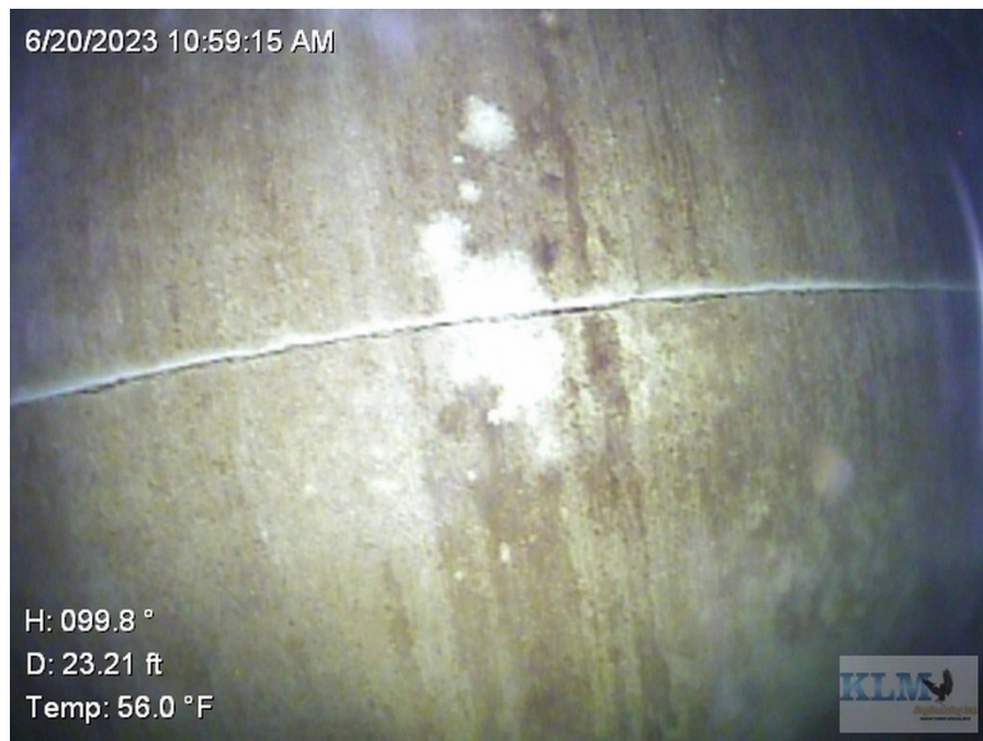
Photo No. 16 Shell coating conditions
