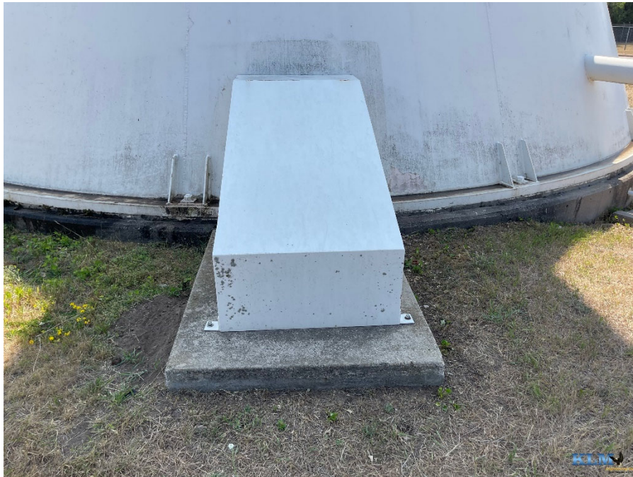
Photo No. 57 Base cone conditions
