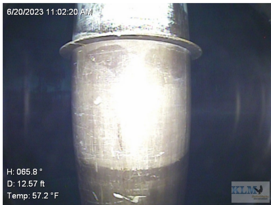
Photo No. 12 Drywell tube conditions
