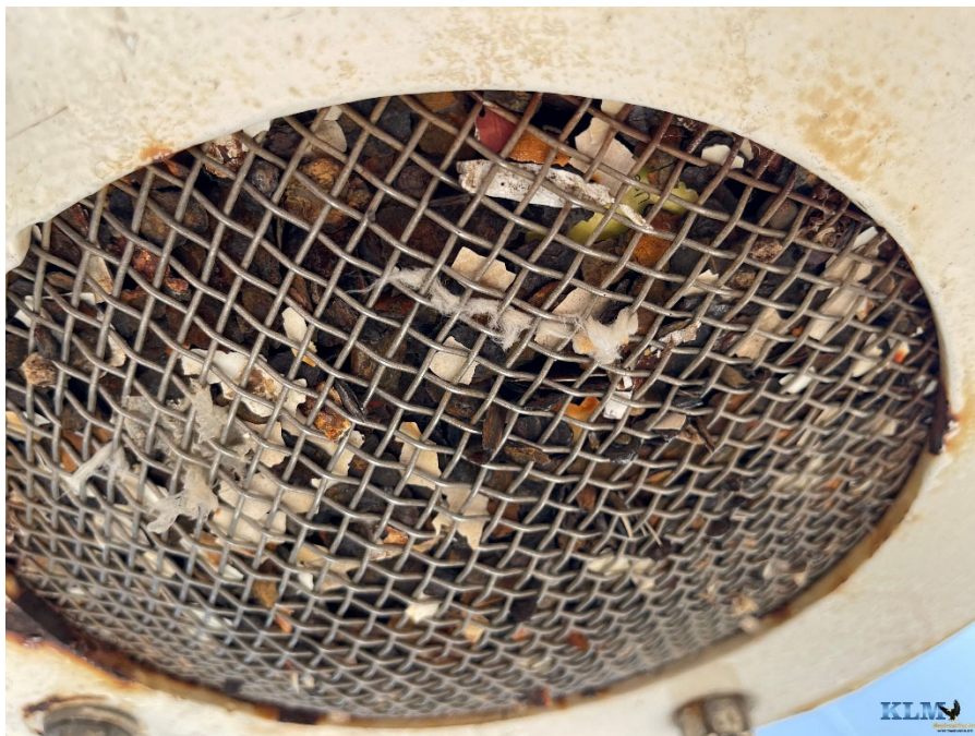
Photo No. 60 Condition of overflow pipe screen
