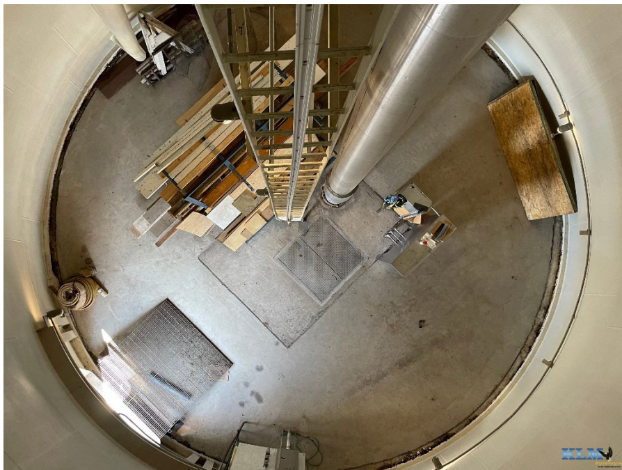
Photo No. 36 View of tower base
