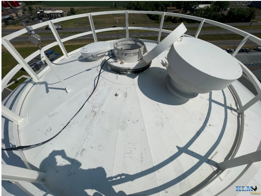
Photo No. 43 View of roof
