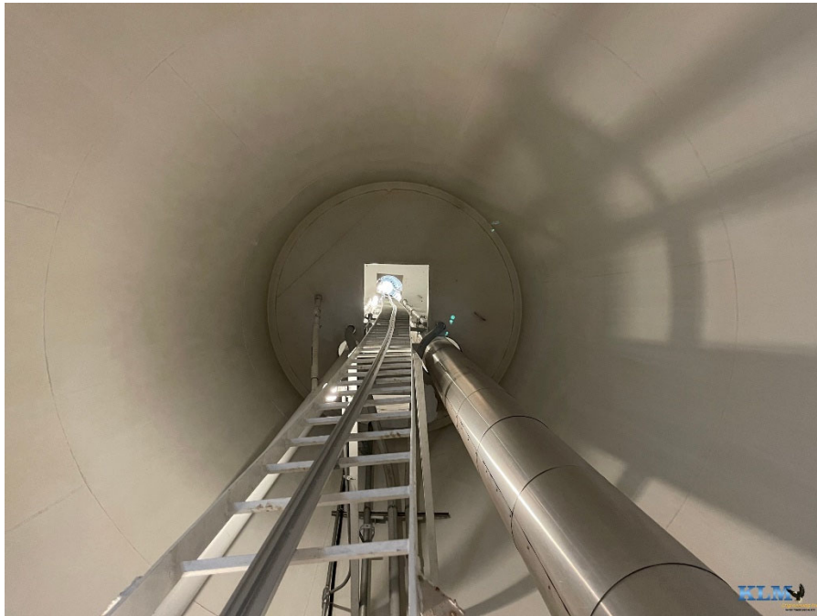
Photo No. 37 Base cone conditions looking up at underside of bottom landing
