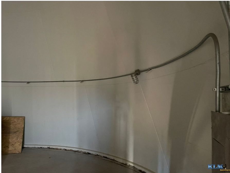
Photo No. 39 Base cone conditions
