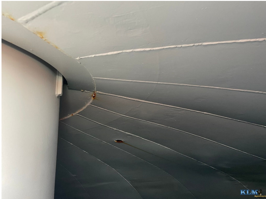
Photo No. 5 Roof conditions
