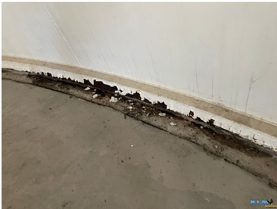
Photo No. 40 Base plate conditions
