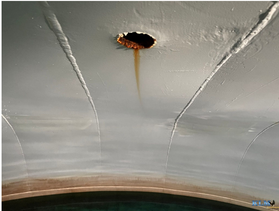
Photo No. 9 Roof condition with rigging coupling visible
