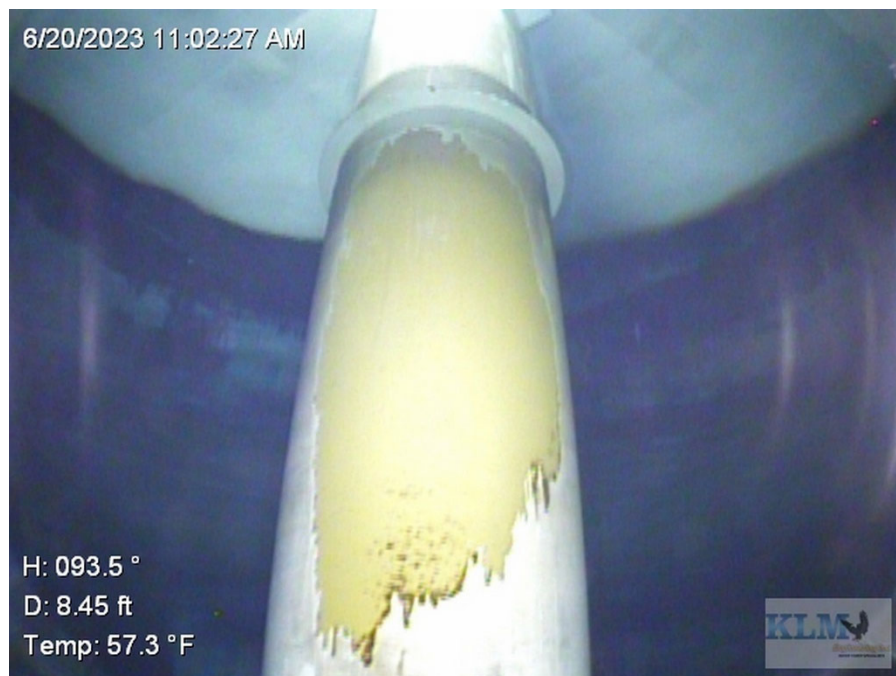
Photo No. 11 Drywell tube conditions below HWL
