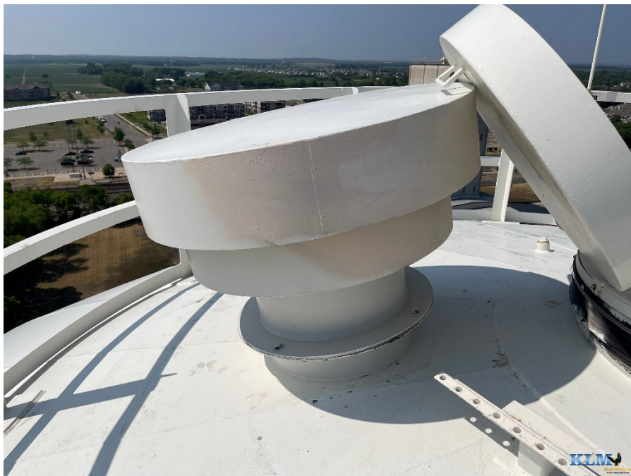
Photo No. 46 Finial vent
