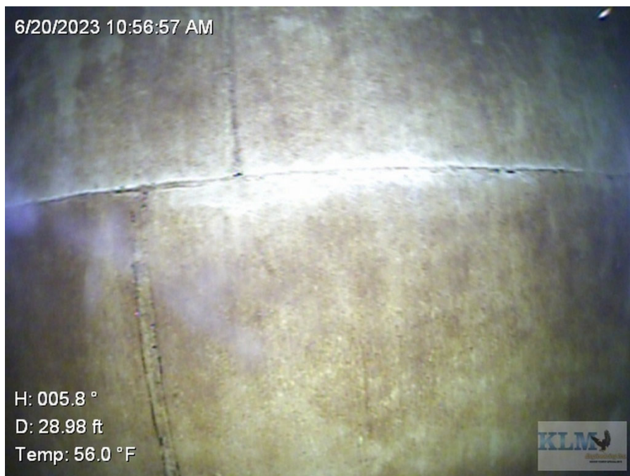
Photo No. 19 Shell coating conditions
