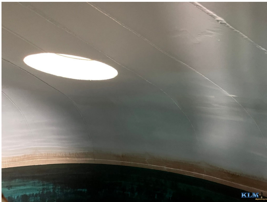
Photo No. 8 Roof conditions with ventilation manway visible
