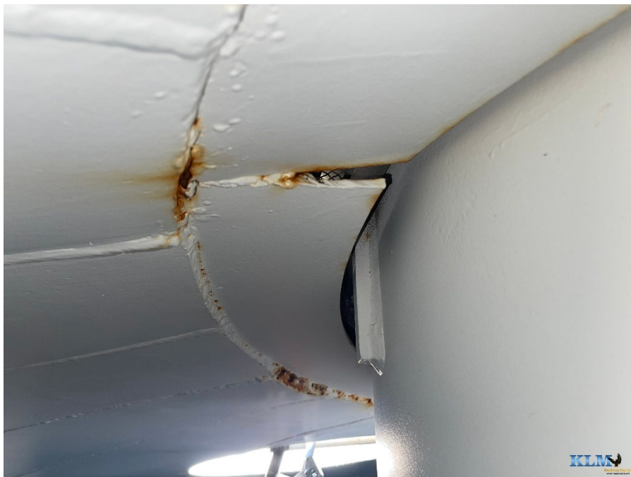
Photo No. 4 Interior roof conditions
