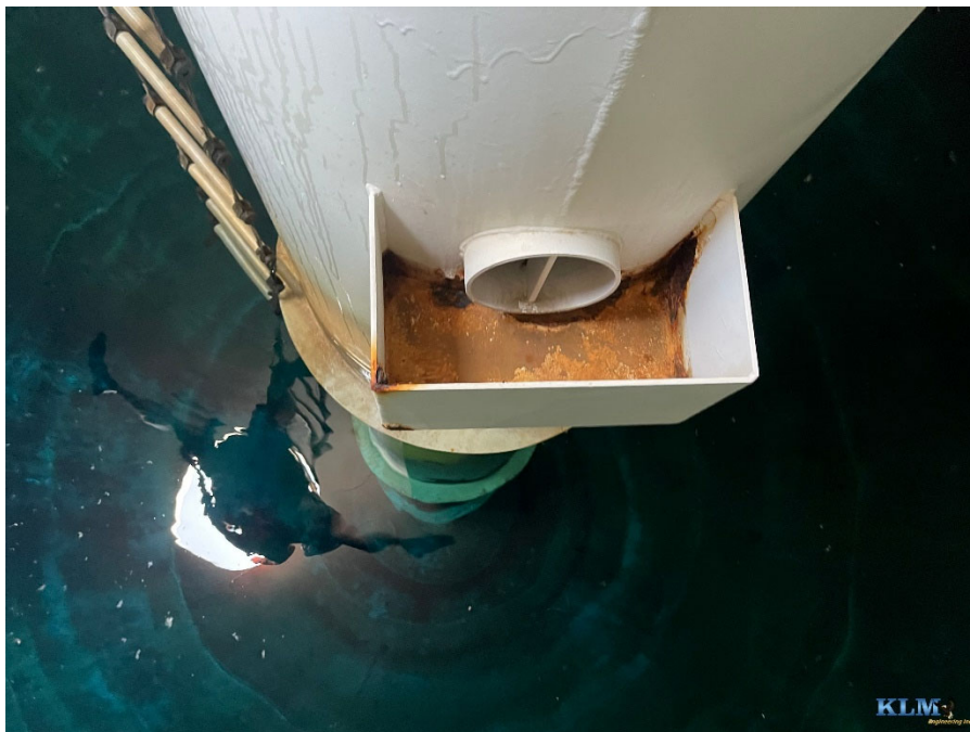
Photo No. 10 Overflow weir box
