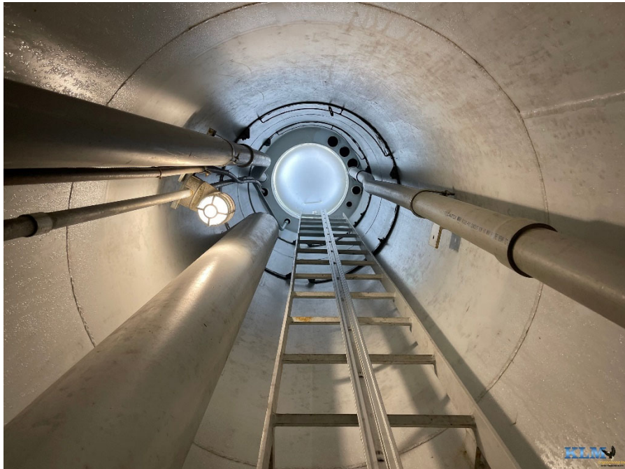
Photo No. 27 Drywell tube conditions
