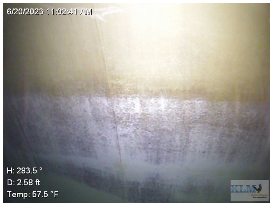
Photo No. 13 Shell coating conditions
