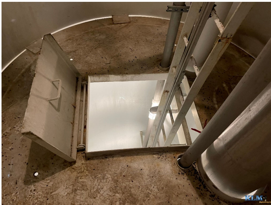
Photo No. 32 Top landing conditions
